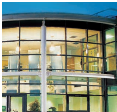
Electric power distribution
